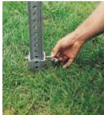
**2** Attach the sign to the post at the desired height using drive rivets or bolts.
